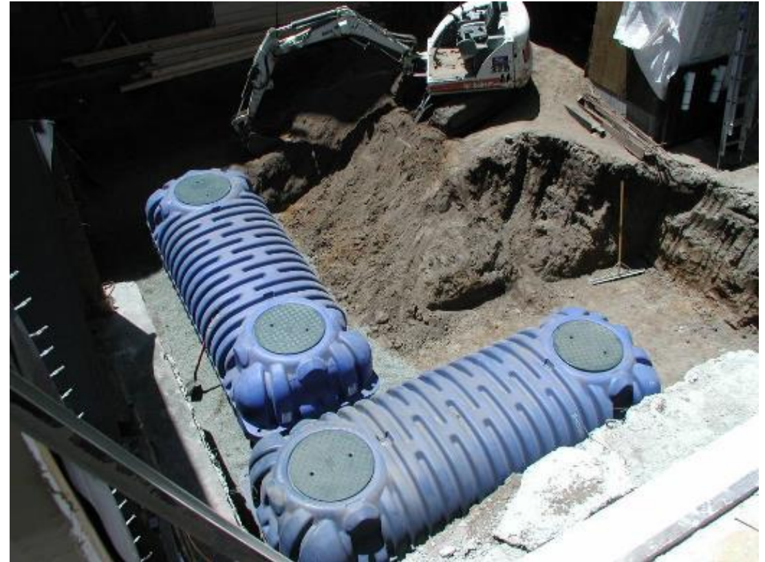
Cisterns installed underground
