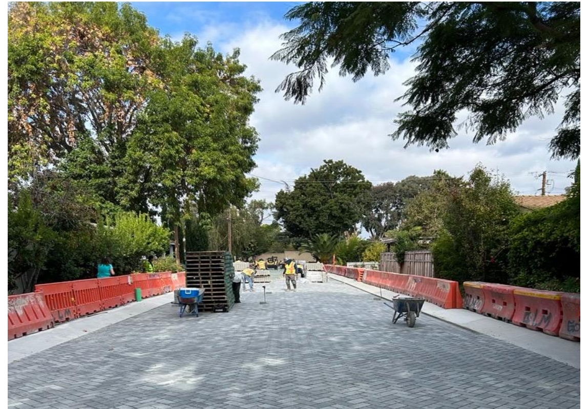
Permeable Interlocking Concrete Pavers (San Jose)
