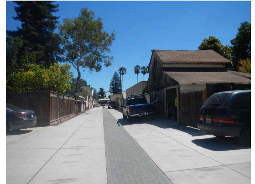
Martha Gardens Green Alleys Project, City of San José
