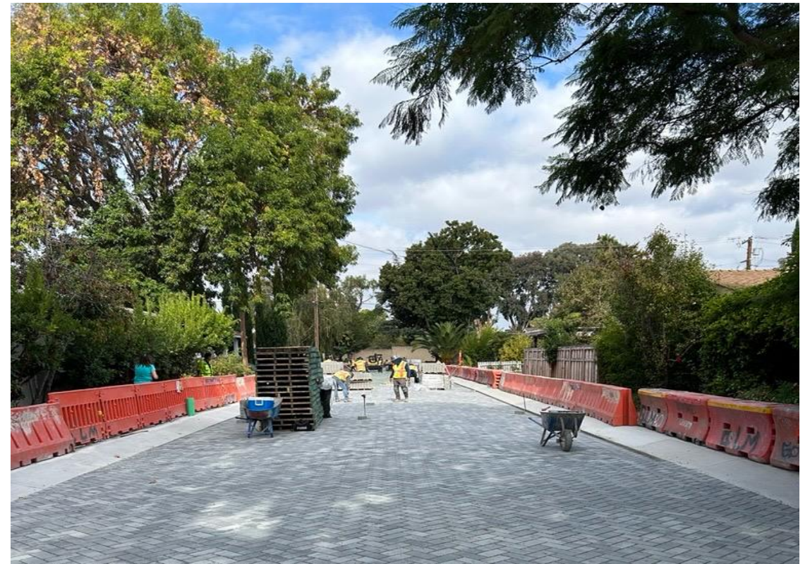
Permeable Interlocking Concrete Pavers (San Jose)
