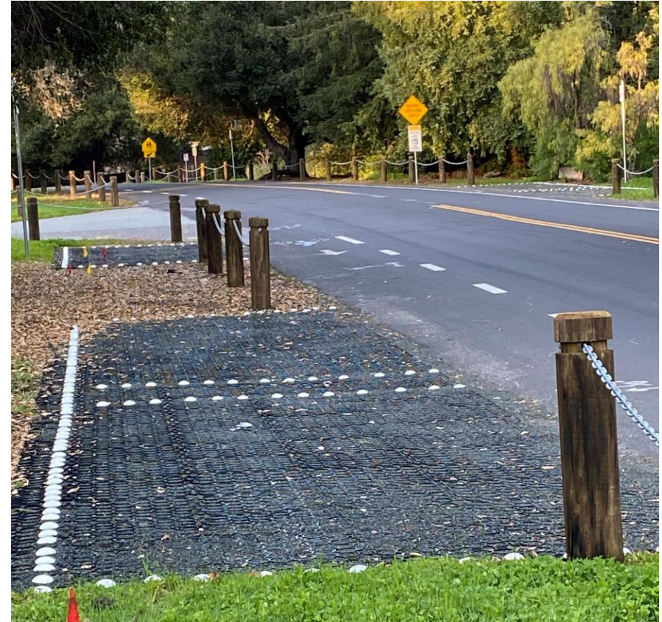
Grid Supported Gravel Pavement (Stanford)
