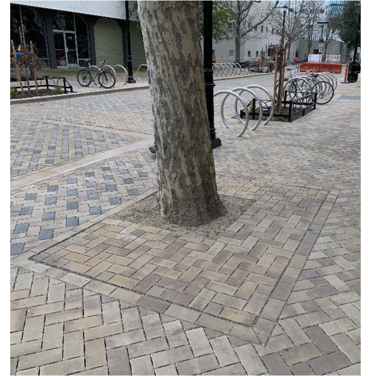
Tree Well Filter/ Pervious Pavement
