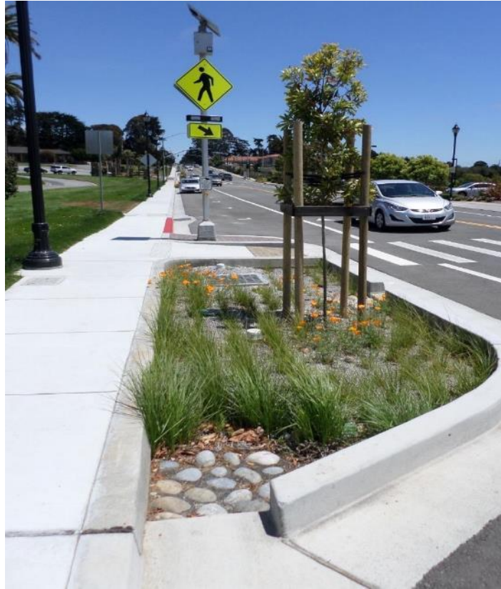
Stormwater Curb Extension
