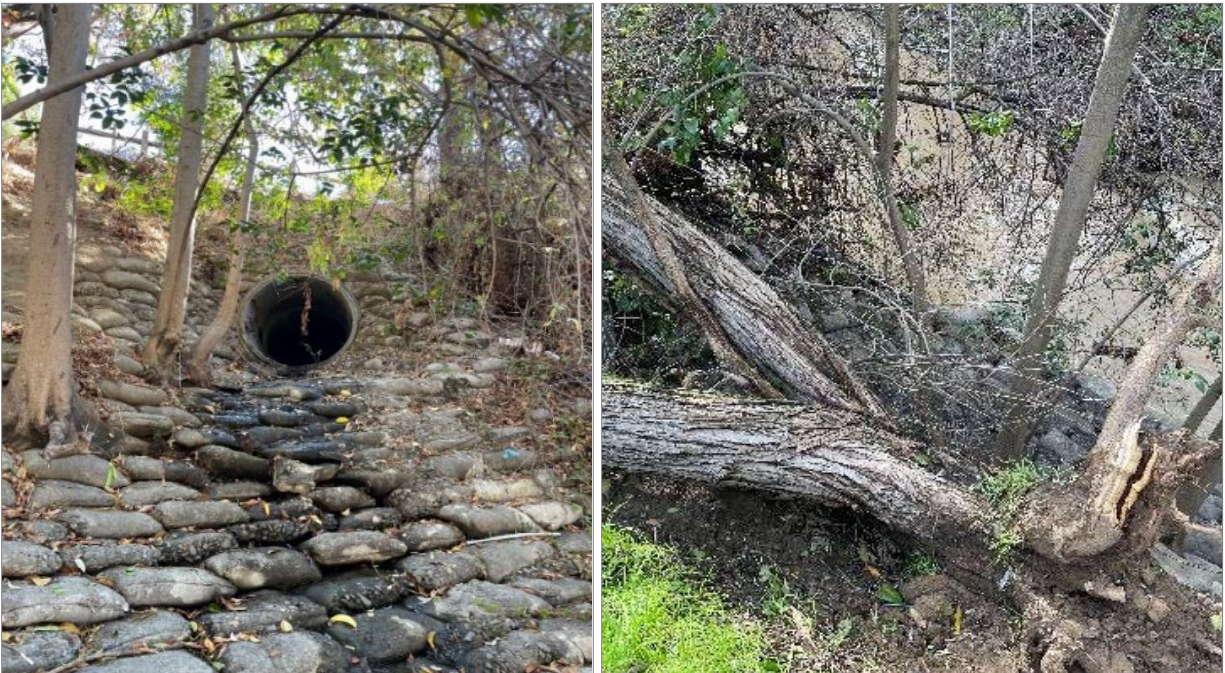
Figure SC-5. Outfall above Stevens Creek, City of Mountain View
