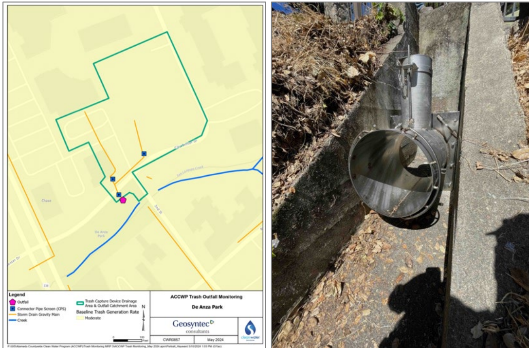
Figure AC-4. AC-CYCTR outfall, with the NetTech™ monitoring device, located on the north bank of San Lorenzo Creek, City of Hayward
