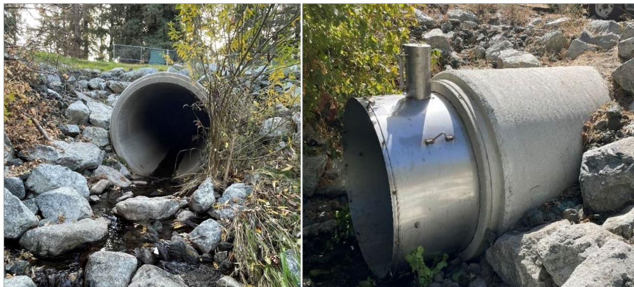
Figure SC-6. Outfall above Coyote Creek, City of San Jose
