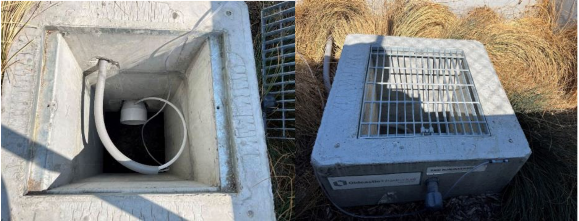
Figure 3.4. Effluent measurement device installed within the overflow vault (left), and the in-basin bypass measurement device installed outside the overflow vault (right) at TCM6 at the TopGolf Public Green Streets Project in San José, CA.
