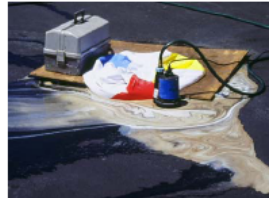
Storm drain inlet is blocked to prevent prohibited discharge. The water must be pumped and disposed of properly.
