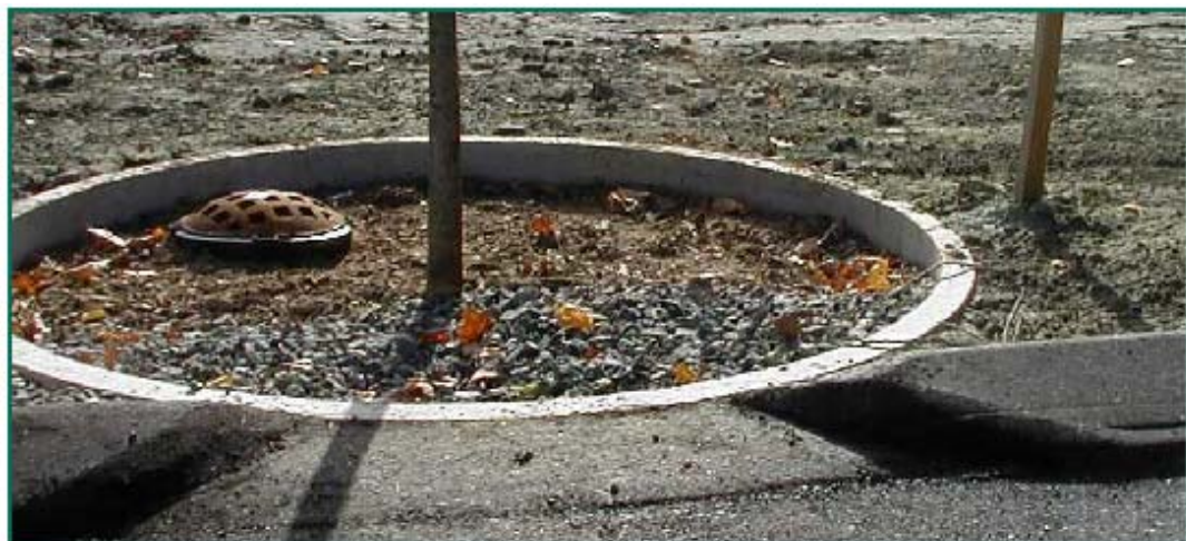
Figure 6-15: Tree Filter with Overflow Bypass. Source: University of New Hampshire Environmental Research Group, 2006
