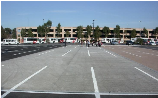
Fig. 8-6 Porous asphalt, pervious concrete and pervious interlocking concrete pavers at Stanford University demonstration project.
