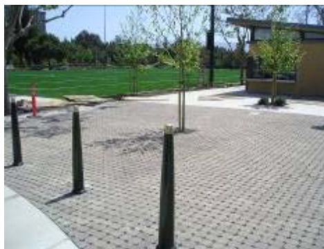
Figure 6-34: Permeable Pavers, Palo Alto
