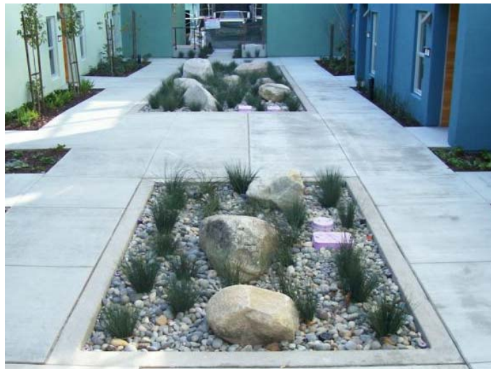
Figure 8-2: Flow-through planter in the City of Emeryville
