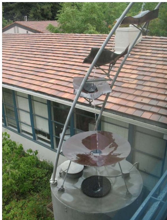
Figure 6-21: Rainwater is collected and used for flushing toilets at Mills College, Oakland.
