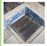
Storm drain inlet on private property
