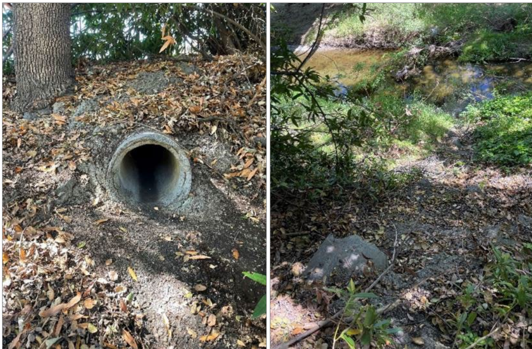
Figure CC-3. Walnut Creek outfall site CC-WC in Civic Park, Walnut Creek
