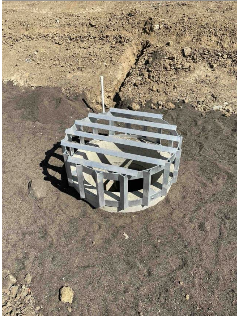
Figure SSA-3. Bioswale overflow pipe in construction (monitoring basket not shown)
