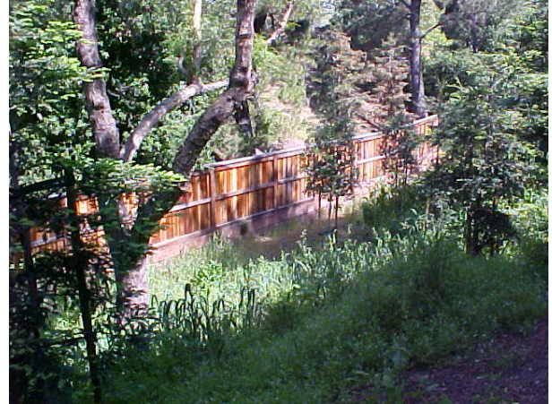
Top view of dry exfiltration basin
