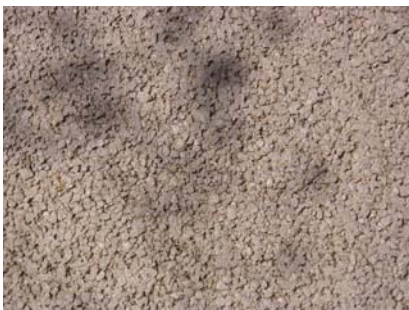
Close-up of pervious concrete
