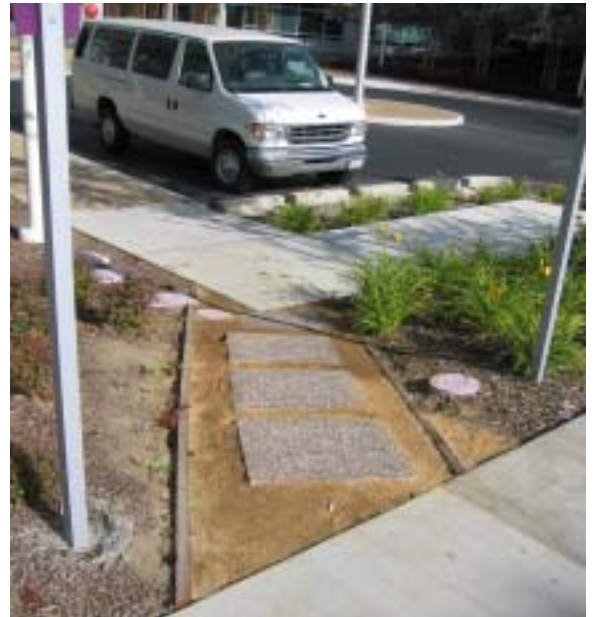
Pervious walkways used between concrete sidewalks.
