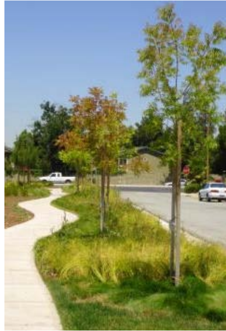
Runoff from surrounding impervious areas flows to vegetated bioswale.
