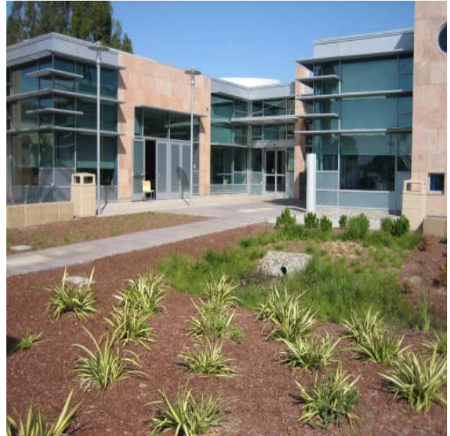
Roof runoff is directed to retention pond for natural treatment of stormwater.
