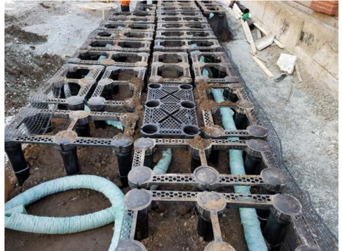
Distribution pipe shown within ponding depth
