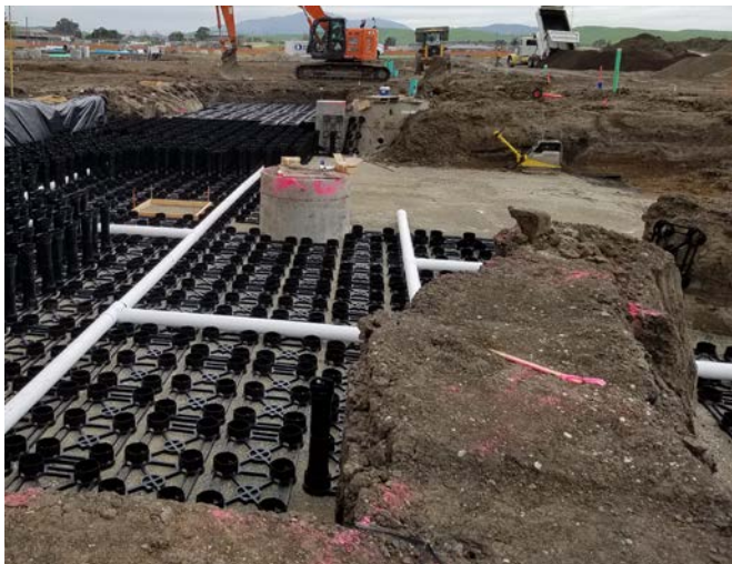
Underdrain being installed at base of system
