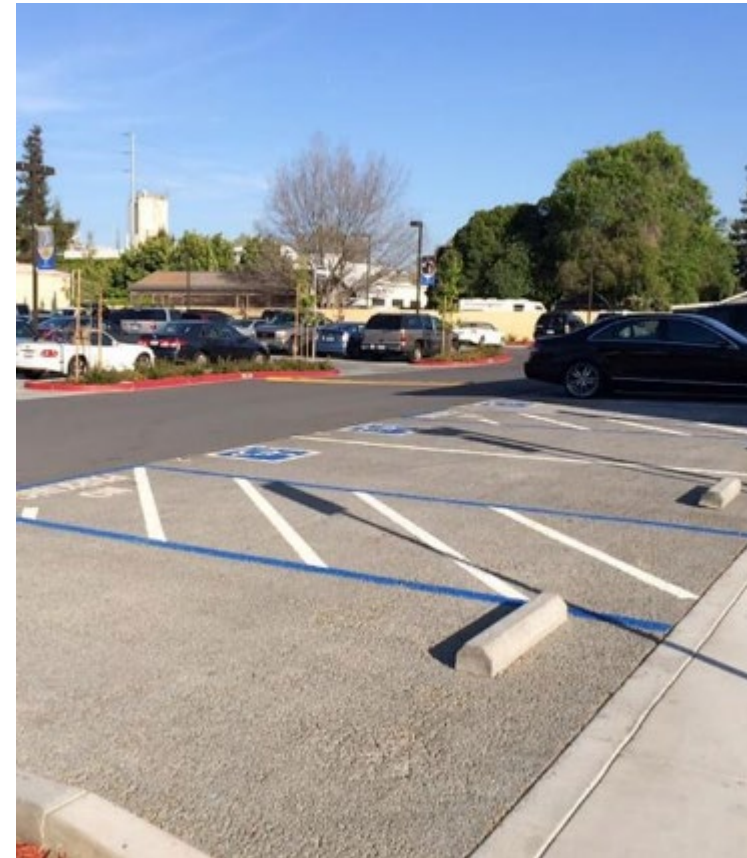
Pervious Concrete Parking Stalls (San Jose, CA)
