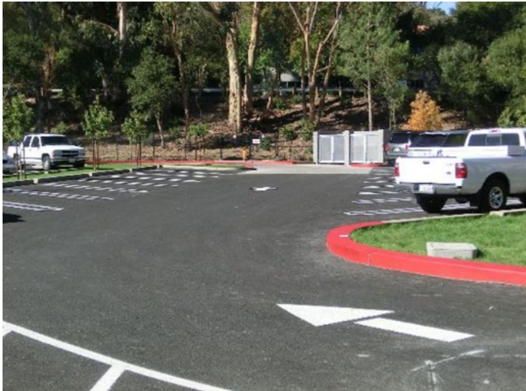
Pervious Asphalt Parking Lot (Los Gatos, CA)
