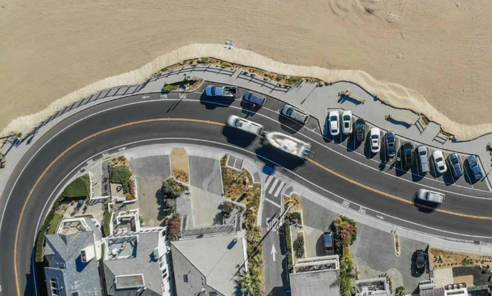
Pictured: Twin Lakes Beachfront Improvements, Santa Cruz, CA
