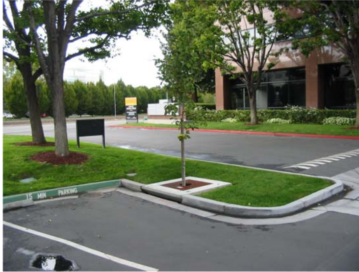
Figure 6-17: Proprietary tree well filter at an office building in San José. Photo: City of San José.
