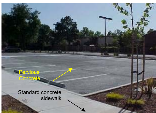
Figure 6-32: Parking Lot with Pervious Concrete, San José
