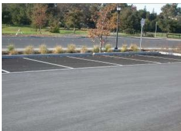
Figure 6-33 Porous Asphalt Parking Lot, Stanford
