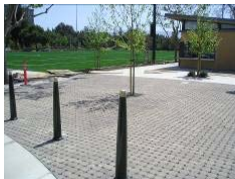
Figure 6-34: Permeable Pavers, Palo Alto
