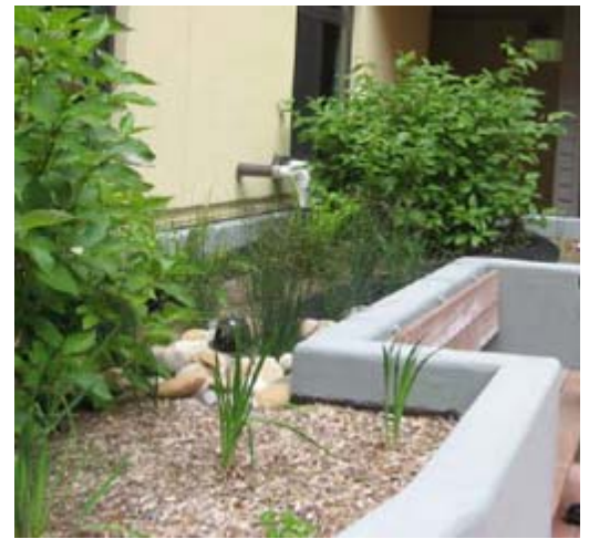
Figure 6-13: The same planter as shown in Figure 6-12, after vegetation has matured and partially conceals the half-buried pipe from view (Source: San Francisco Estuary Partnership).
