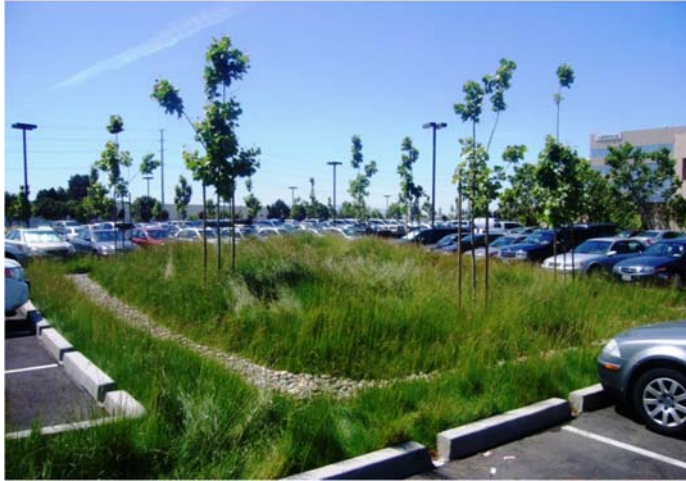
Figure 6-1: Bioretention area in office building parking lot in San José. Source: City of San José.
