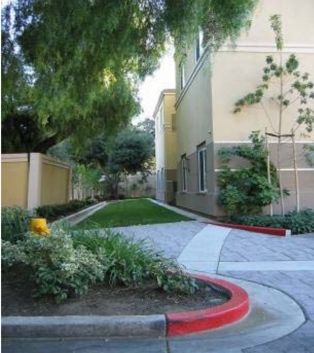
Figure 6-40: Turf block fire access at the Residence Inn in Los Altos
