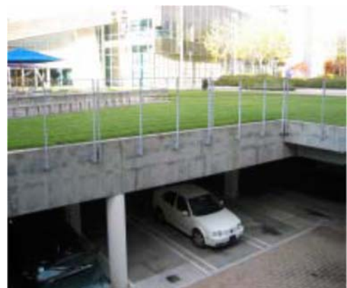
Figure 6-31: Intensive Green Roof at Google, Mountain View.
