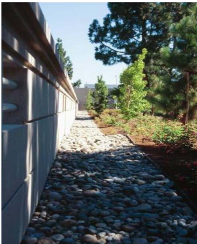
Figure 6-18: Infiltration trench next to parking structure, Palo Alto. Photo: EOA, Inc.
