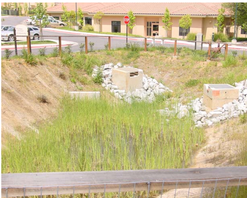
Figure 6-25: Extended detention pond. Source: City of Saratoga
