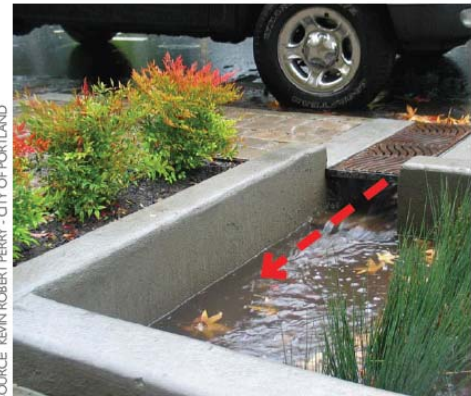
Figure 5-11: A grated curb cut allows stormwater to pass under a pedestrian walkway to the stormwater facility.
