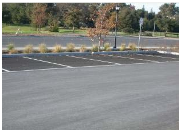
Figure 6-33 Porous Asphalt Parking Lot, Stanford
