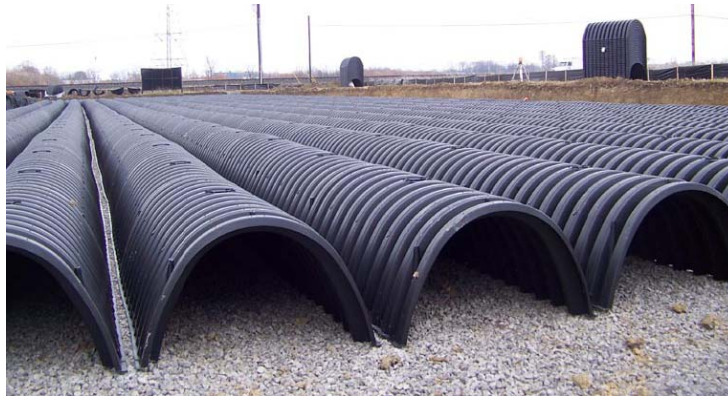
Figure 6-20: Photo of subsurface retention/infiltration system installation under a parking lot. Source: CONTECH Engineered Solutions.
