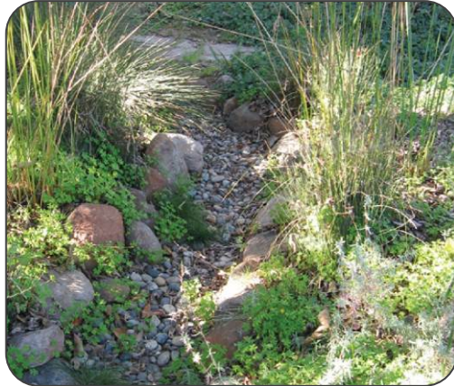
Dry creek infiltrates and conveys runoff.
