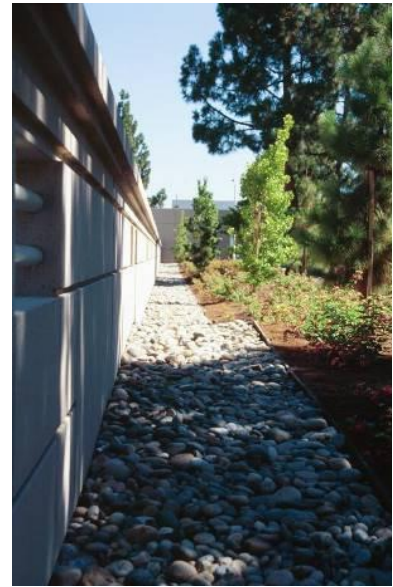
Figure 8-4: Infiltration Trench at former Agilent site, Palo Alto
