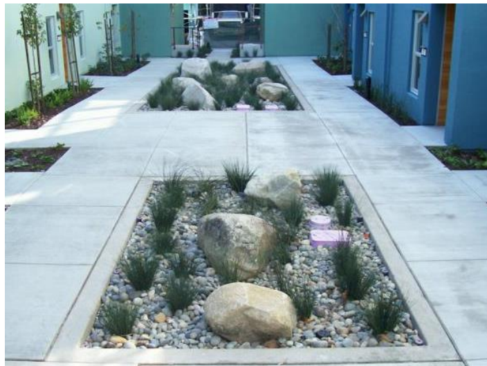
Figure 8-2: Flow-through planter in the City of Emeryville
