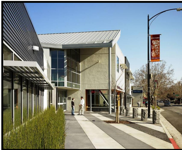
Figure 8-3: Pervious asphalt directs water to an enlarged tree well filled with engineered 'structural soil', San José.
