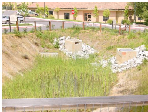
Figure 8-5: Detention pond at a retirement center in Saratoga
