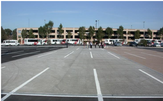
Fig. 8-6 Porous asphalt, pervious concrete and pervious interlocking concrete pavers at Stanford University demonstration project.
