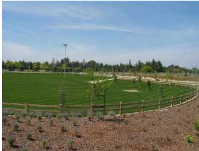
Figure 7-5: Example of a multi-purpose detention facility for HM control in San Jose.
