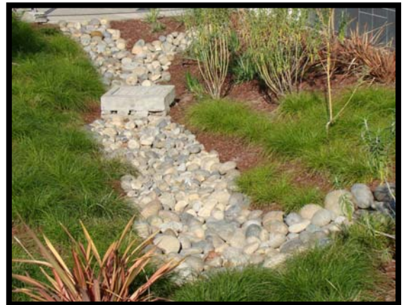
Figure 5-1: Cobbles in this stormwater treatment measure in San José help prevent erosion.
