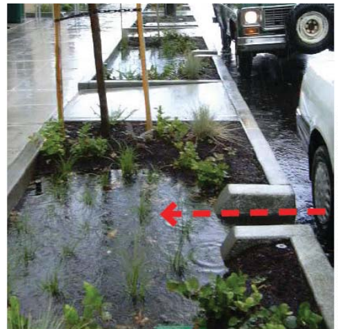
Figure 5-5: The side wings of this standard curb cut help retain the side slope grade on each side of the curb cut opening.
