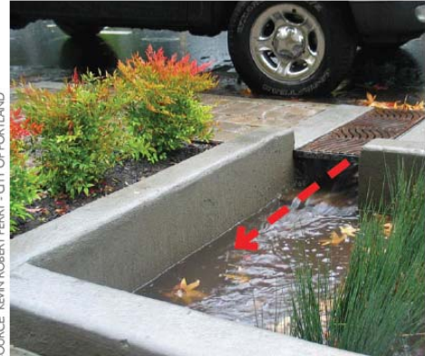
Figure 5-11: A grated curb cut allows stormwater to pass under a pedestrian walkway to the stormwater facility.
