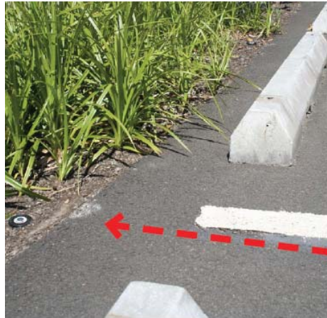
Figure 5-8: Stormwater runoff enters the stormwater facility through the 3-foot space between these wheelstops. The design could be improved by providing more of a drop in grade between the asphalt and landscape area.
