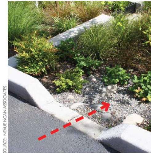
Figure 5-2: This standard curb cut at parking lot rain garden has 45 degree chamfered sides.
