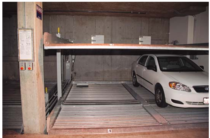
Figure 4-7: Parking Lifts in Parking Garage, Berkeley
