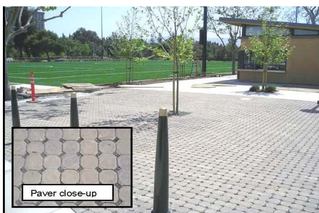
Figure 4-6: Pervious paving at Mayfield Soccer Field in Palo Alto.
