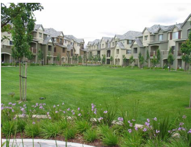
Figure 3-8: This landscaped area in San José also functions as a stormwater treatment area.
