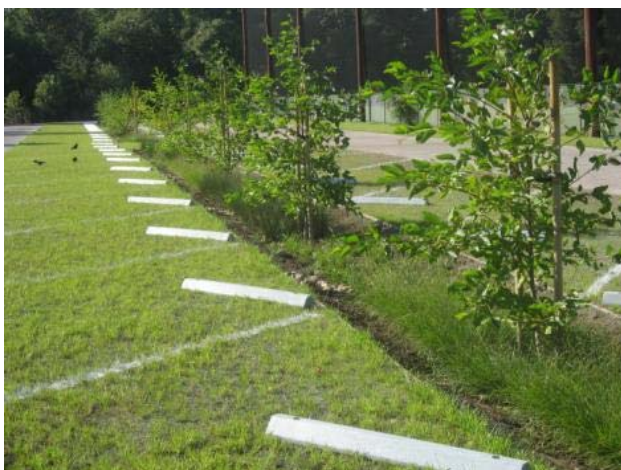
Figure 3-5: Stevens Creek Corridor Park in Cupertino includes turf block pavers in parking lot.
