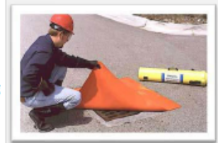
Protect the storm drain
