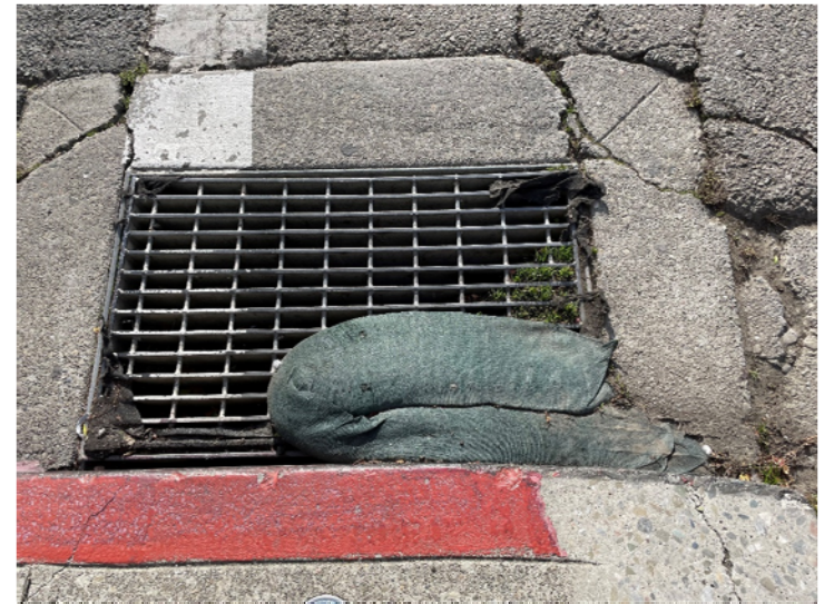
Abandoned filter bag and fiber roll months after road repair completed
