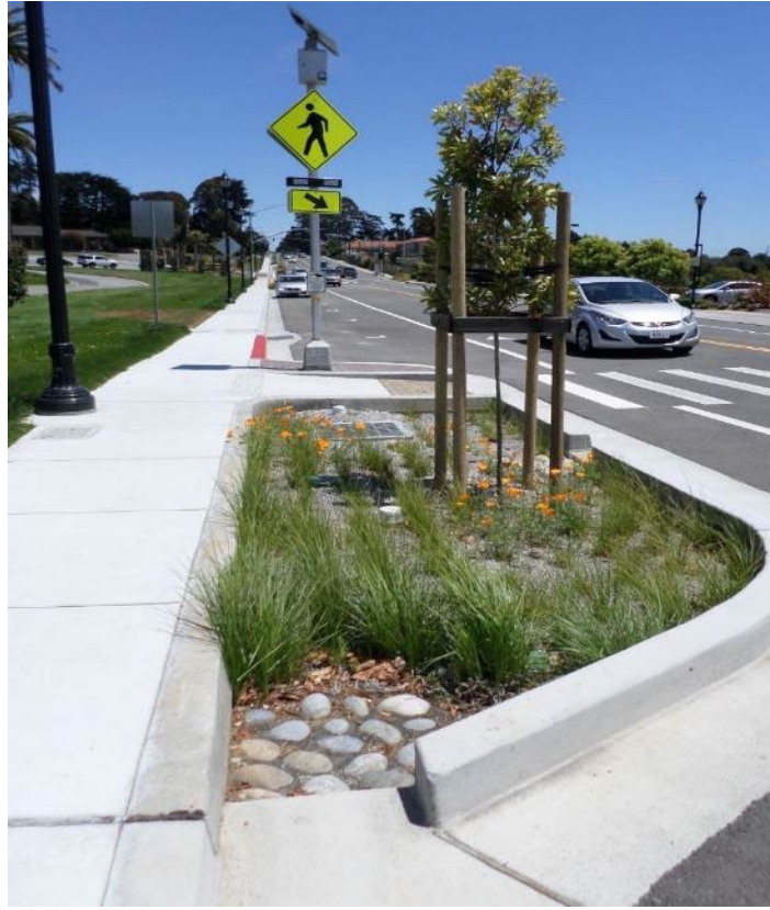
Stormwater Curb Extension
