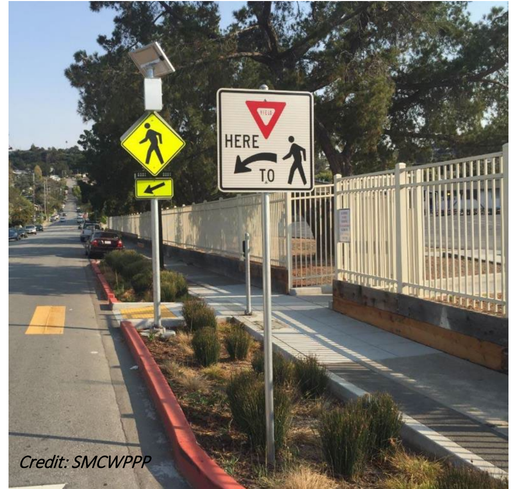
Stormwater curb extension in Safe Routes to School improvements (San Mateo, CA)
