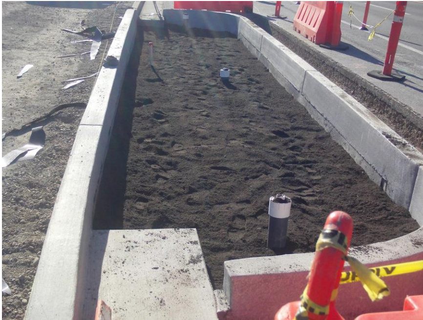
April 26, 2020 – Bioretention soil added
