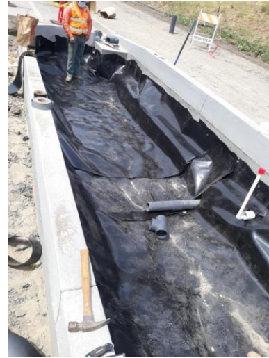
April 20, 2020 – Geomembrane and perforated pipe
