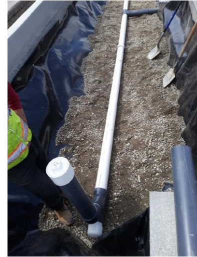
April 20, 2020 – Geomembrane and perforated pipe
