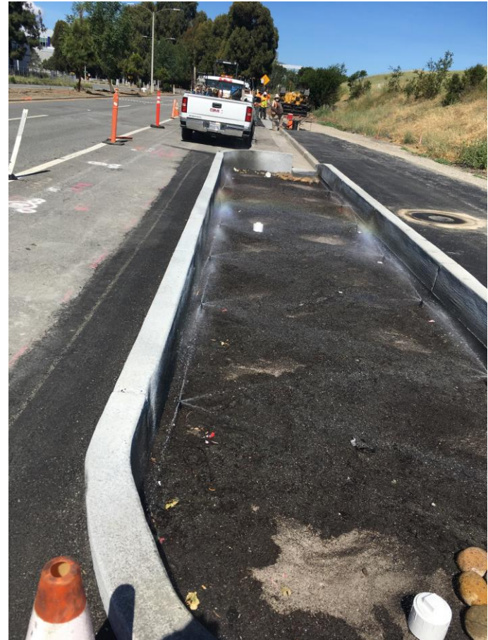
May 20, 2020 – Irrigation installed
