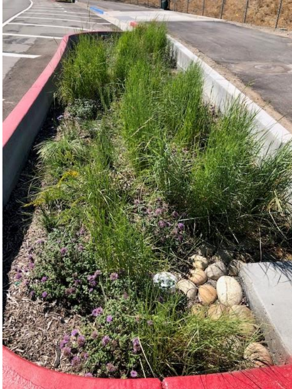
June 2020 – Completed bioretention areas
