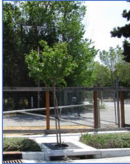
TREE WELL FILTER
