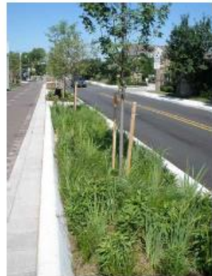
6' BIO SWALES - TREES, SMALL SHRUBS/ GROUND COVER & TALL GRASSES
