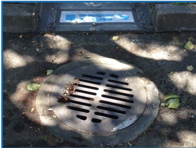
Cleaned and newly labeled storm drain inlets.
