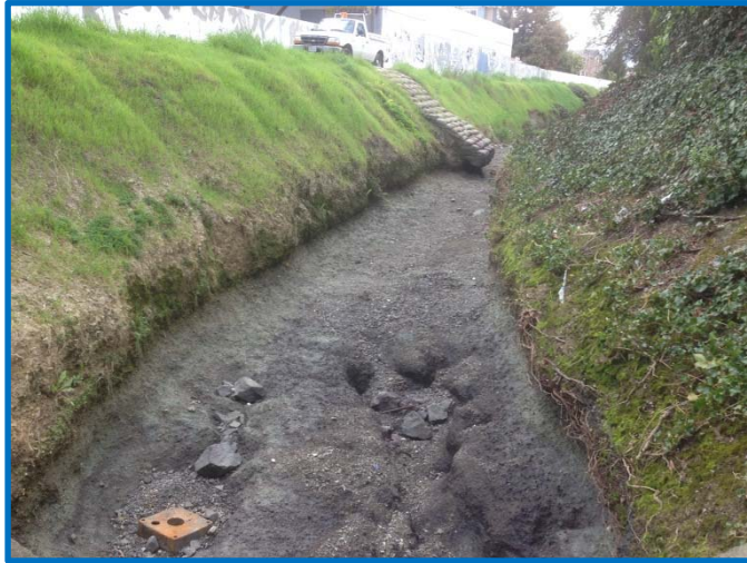
Initial Cleanup effort by Santa Clara Valley Water District.
