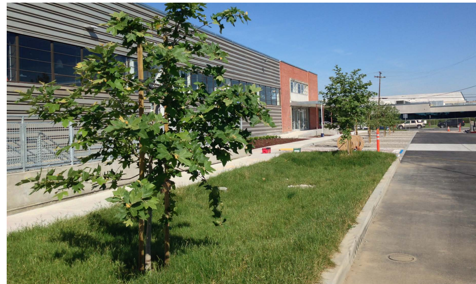
Pervious surfaces and smart, recycled water irrigation system (before & after)
