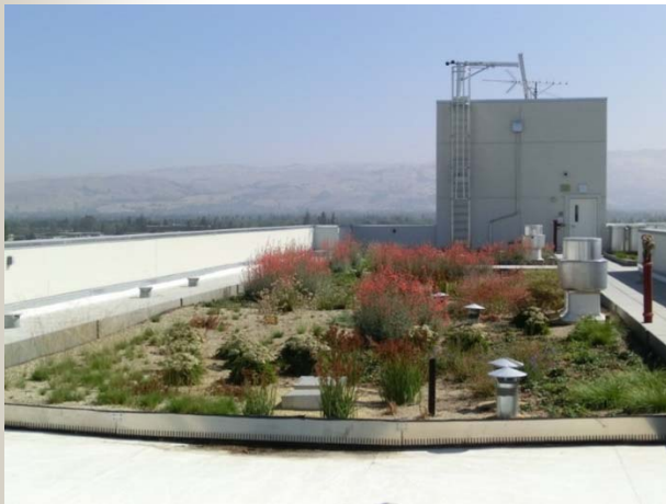
Green Roof at Fourth Street Apartments, San Jose
