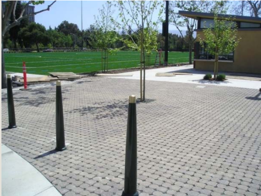
Permeable Pavers, Mayfield Playing Fields, Palo Alto
