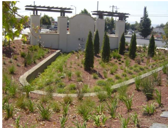
Vegetated Swale and Detention Area Behind Entrance Sign, Modern Ice, San Jose
