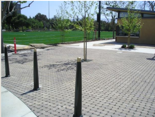
Permeable Pavers, Mayfield Playing Fields, Palo Alto
