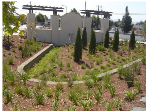
Vegetated Swale and Detention Area Behind Entrance Sign, Modern Ice, San Jose
