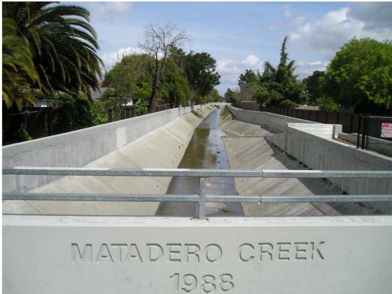
Concrete Lining with Floodwall – Matadero Creek
