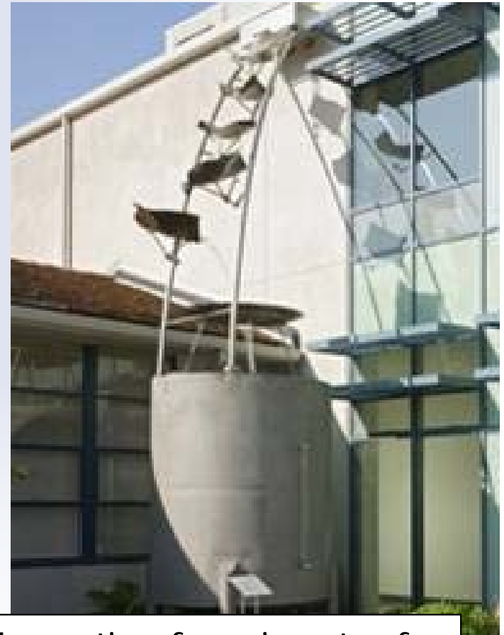
Harvesting for rainwater for indoor toilet flushing
