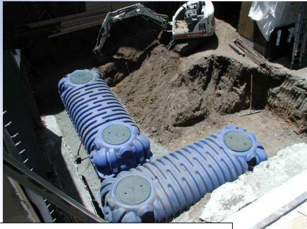
Cisterns installed underground
