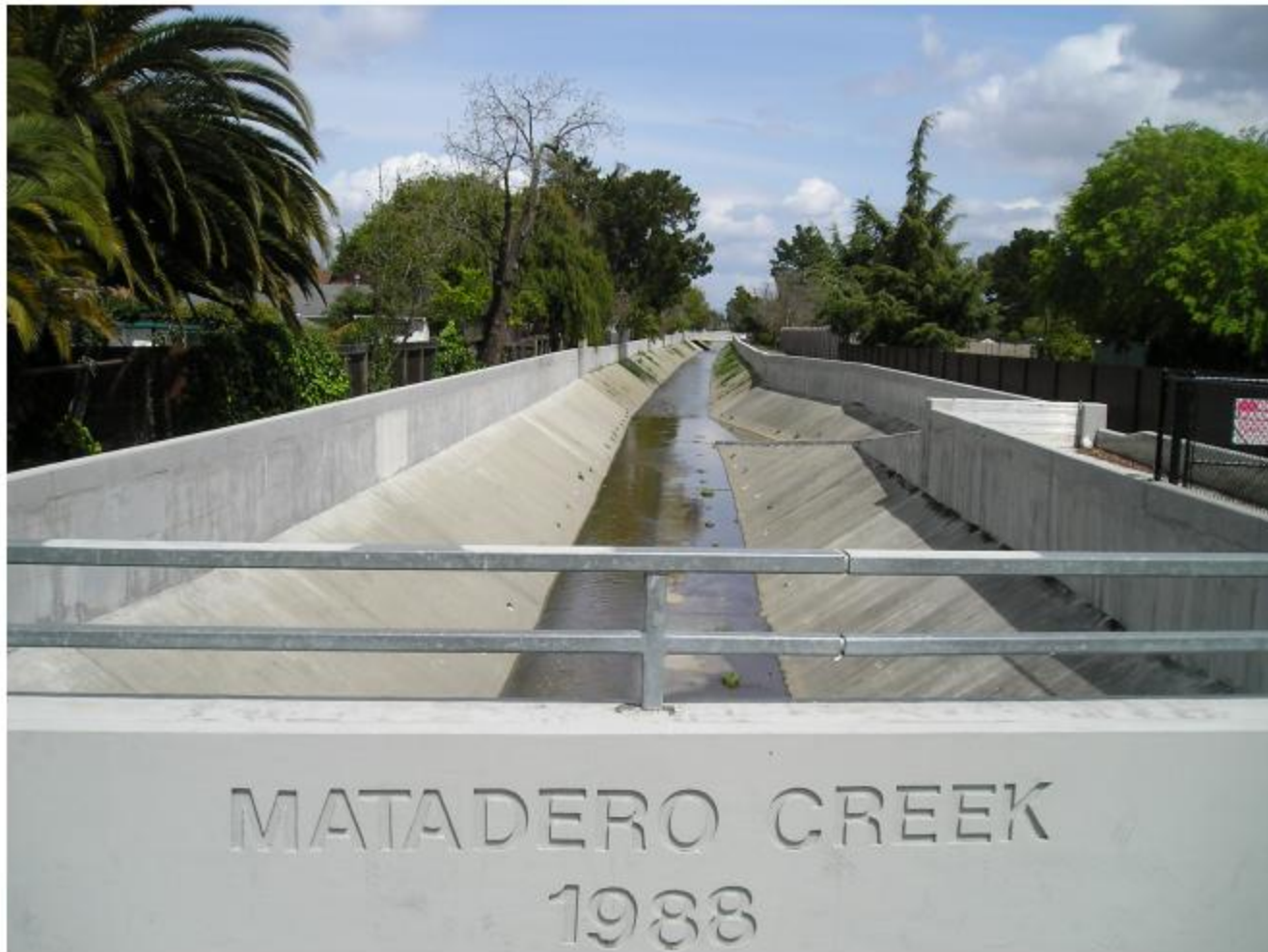
Concrete Lining with Floodwall – Matadero Creek
