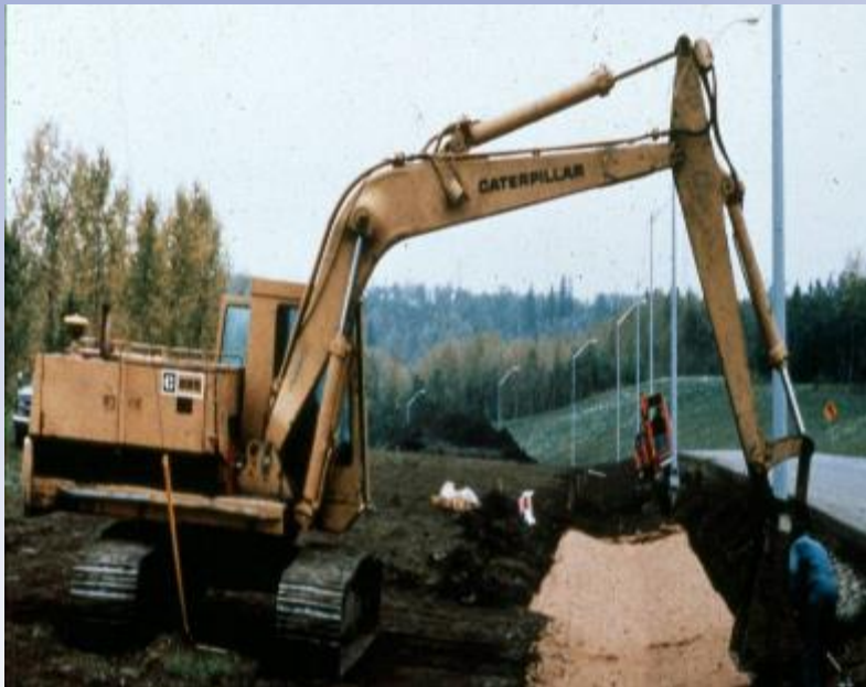
Example of a construction best management practice (BMP)
