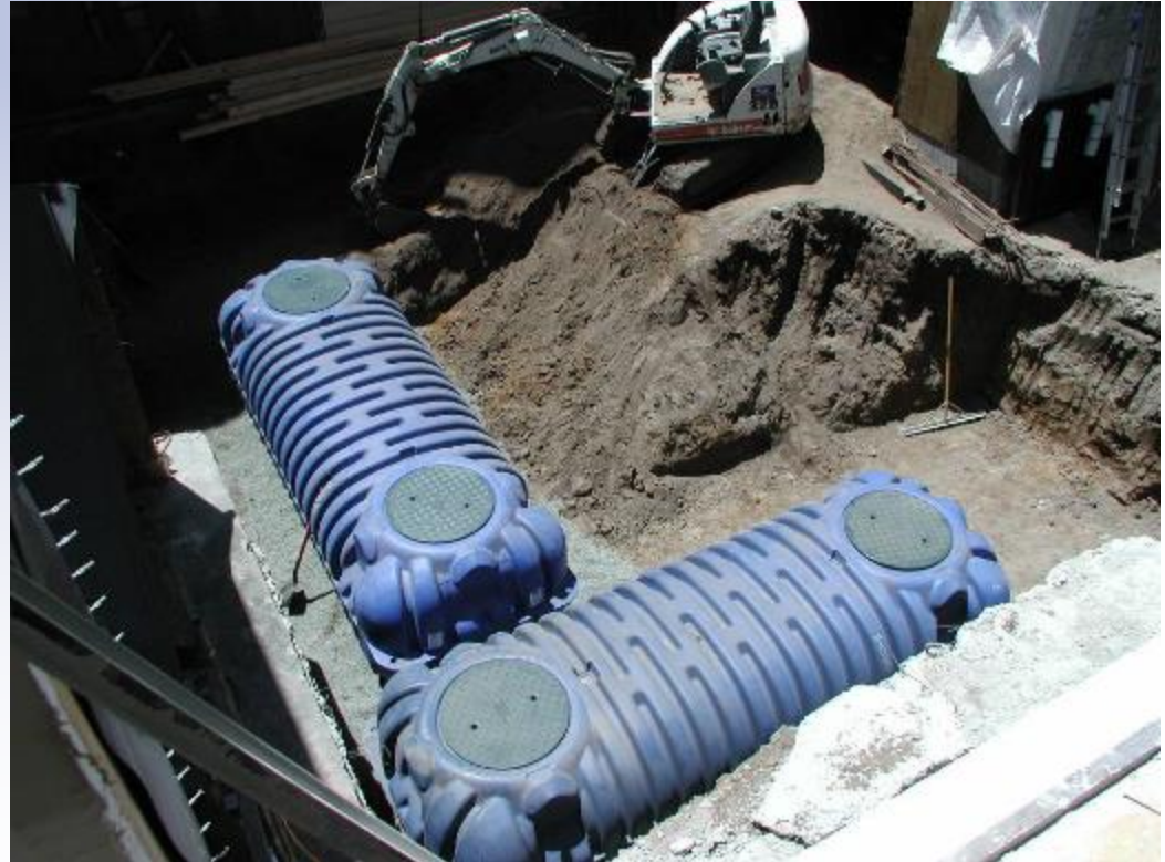
Cisterns installed underground
