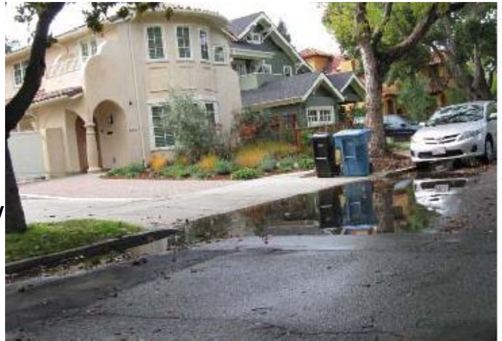
Figure 6-5. Localized ponding before green stormwater infrastructure upgrades in the Southgate Neighborhood. (Credit: Palo Alto.)
