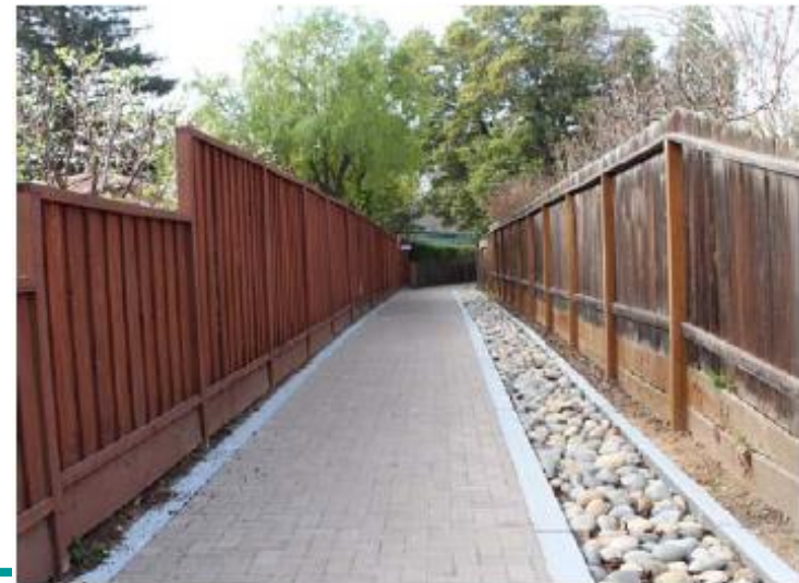
Figure 6-7. A paseo with permeable pavers and an infiltration trench connects Southgate Neighborhood to El Camino Real. (Credit: EOA)
