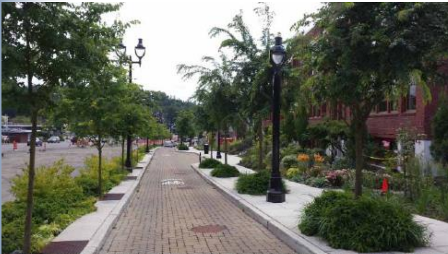
Figure 3-12. One-way, class III bikeway with pervious pavement and Silva Cells for street tree planting in Bothell, WA. (Courtesy of DeepRoot GSI, LLC)
