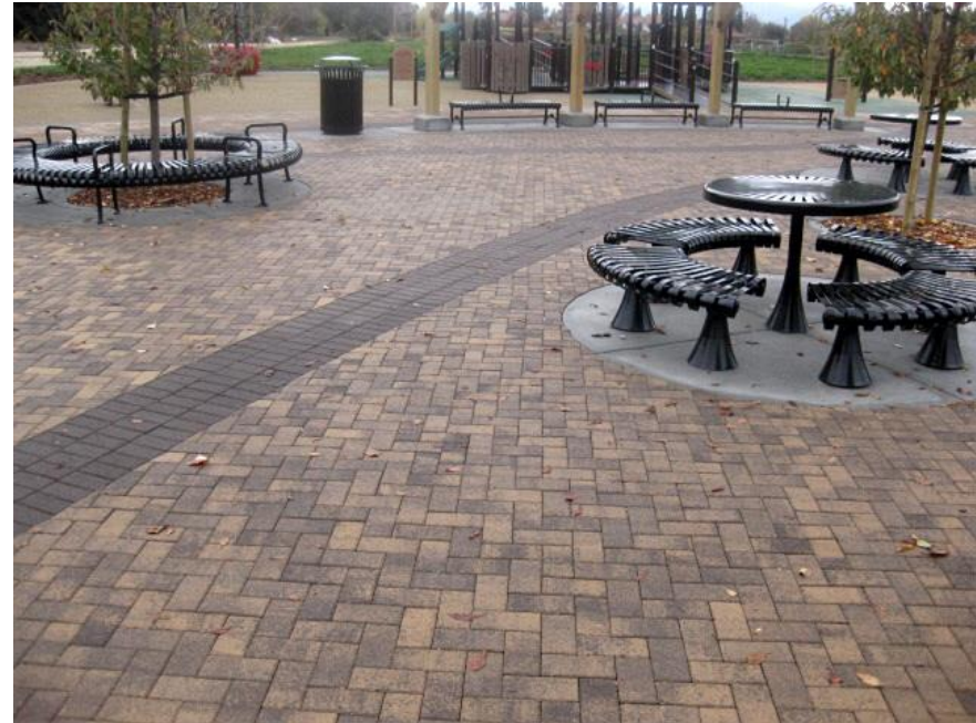
Pervious Pavers, Commodore Park, San Jose
