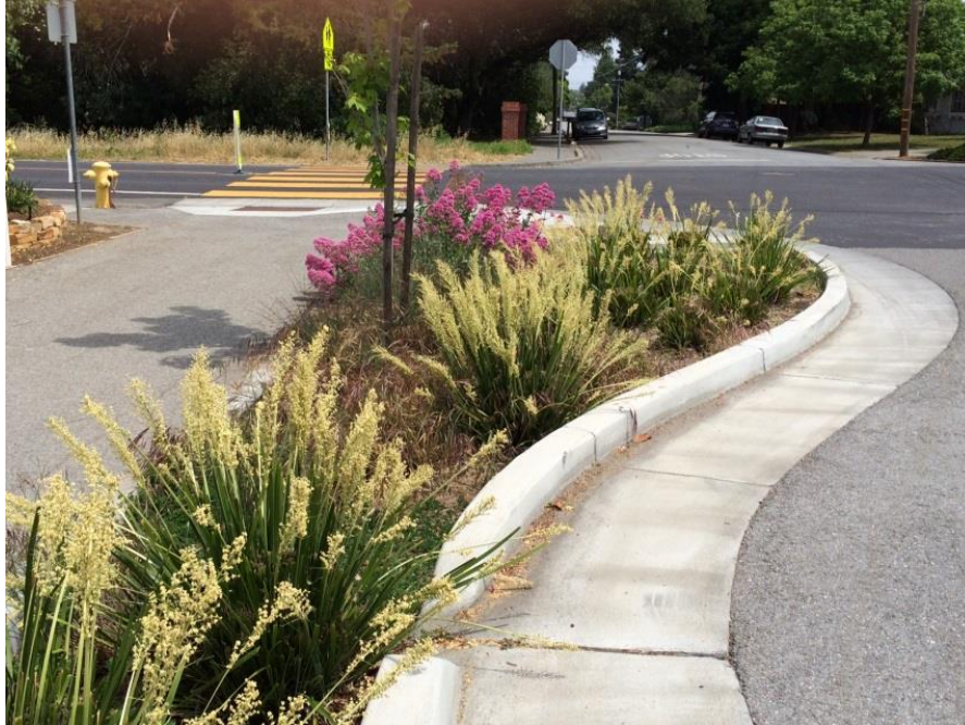
Bioretention area in a curb bulb-out, Rosita Park Neighborhood, Los Altos
