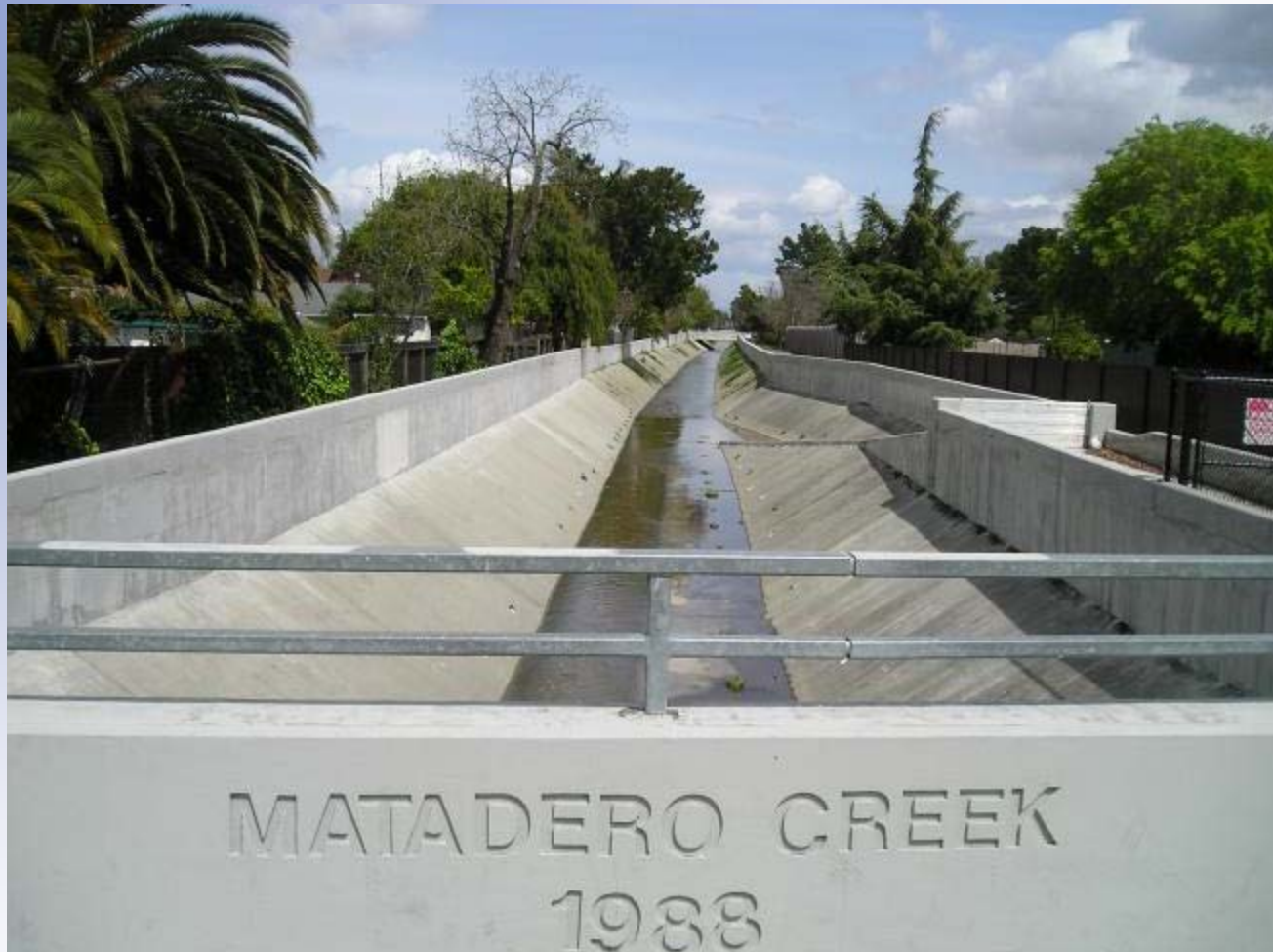
Concrete Lining with Floodwall in Lower Matadero Creek
