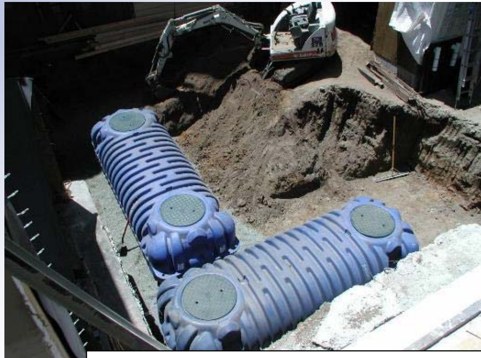
Cisterns installed underground
