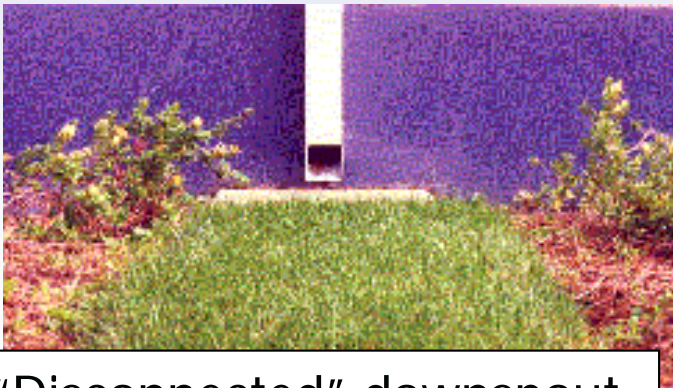
"Disconnected" downspout
